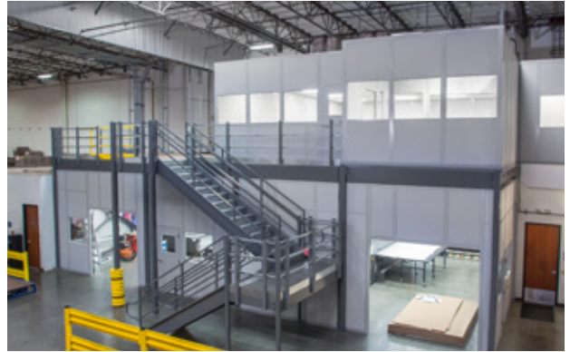
Photo: In-Plant Office Mezzanine
