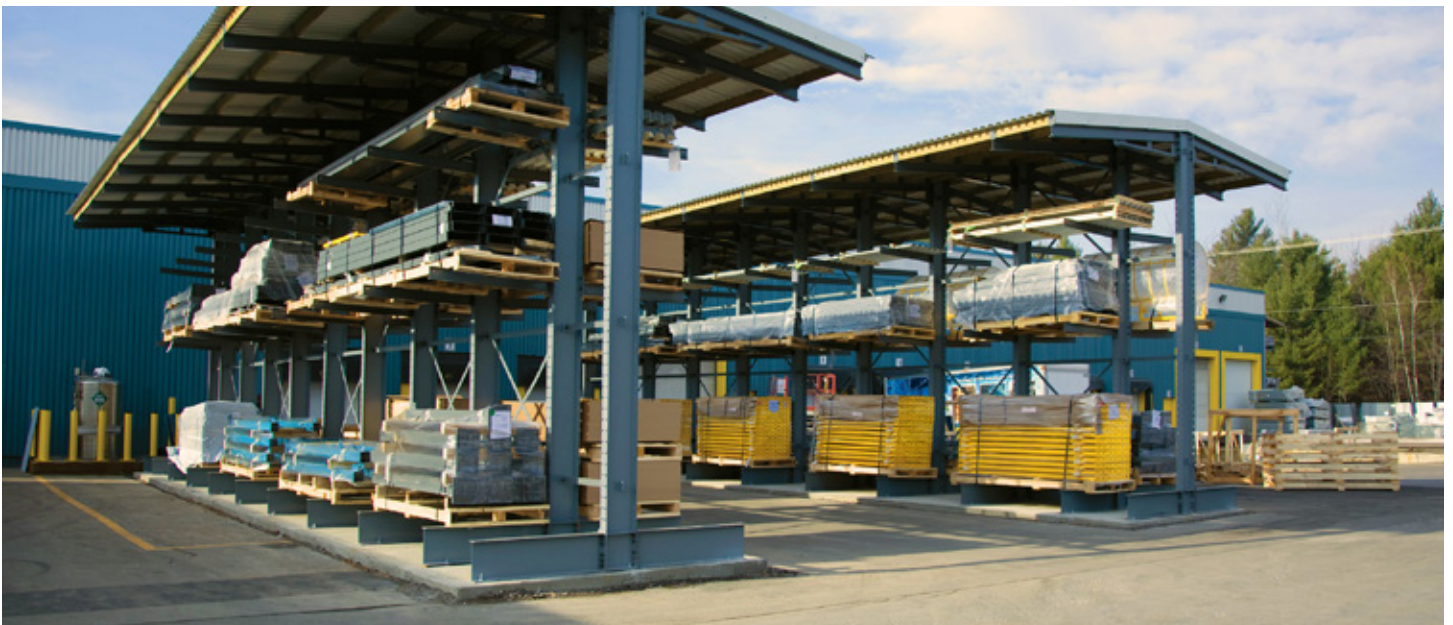
Photo: Four Season Cantilever Roofs
