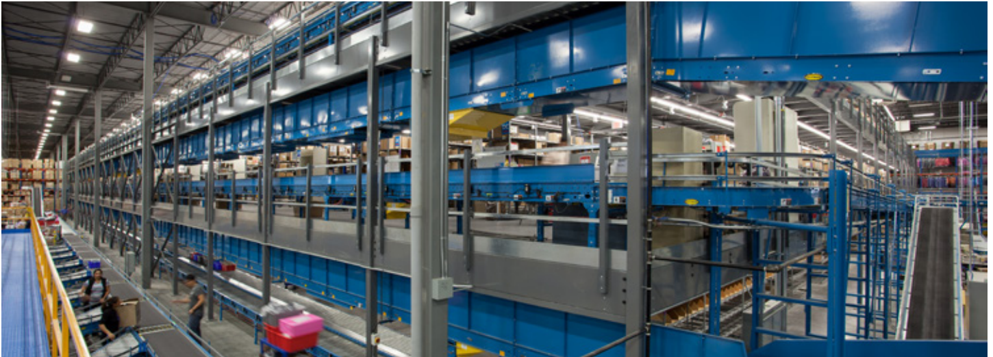
Photo: Conveyor Support Mezzanine
