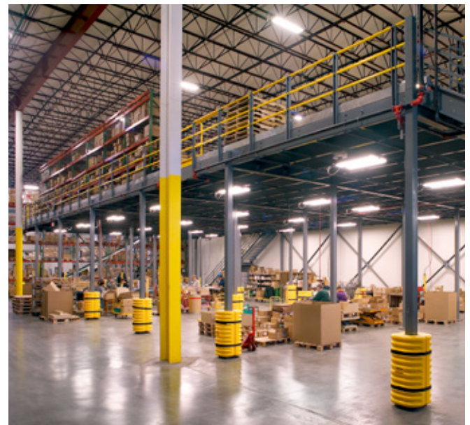
Photo: Warehouse Storage Mezzanine
